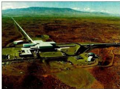
Left: The Hanford Gravitational Wave Interferometric Observatory. The Corner station with one of its 4 km arms extending into the desert is visible, with the perpendicular arm disappearing on the right. Right: Robert Schofield, Ray Weiss and Bill Kells watch the beam monitors in the Hanford control room during one of the LIGO 2 km full-lock acquisitions.
